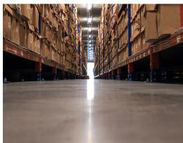
The use of a light-coloured hardener (white or light grey) provides better **reflectivity** and reduces the lighting requirements of a building, consequently saving energy. A DRT Polish final treatment can be applied to increase the brightness and improve the energy performance of the building.
