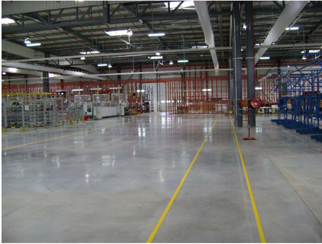
16.500 m 2 concrete based flooring 18 cm with metallic fibres Eurosteel 50/100 and QUALITOP NT HP solution.
