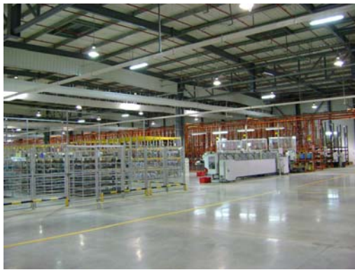
16.500 m 2 concrete based flooring 18 cm with metallic fibres Eurosteel 50/100 and QUALITOP NT HP solution.
