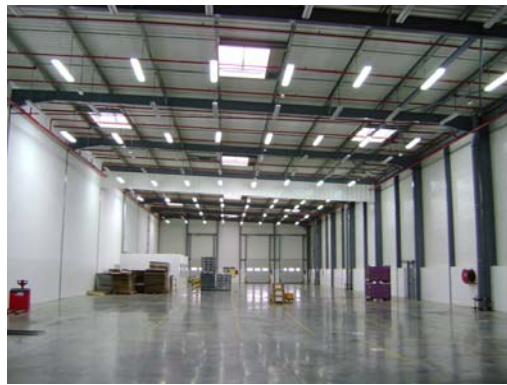
16.500 m 2 concrete based flooring 18 cm with metallic fibres Eurosteel 50/100 and QUALITOP NT HP solution.
