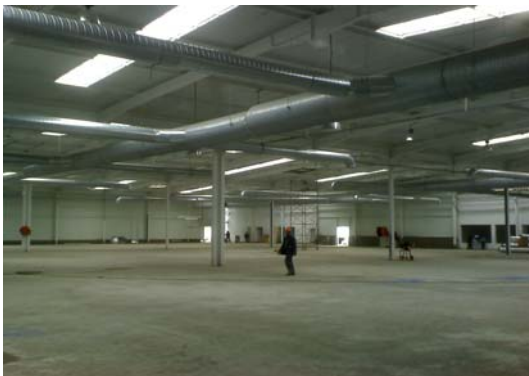
20.000 m 2 concrete based flooring 15 cm with metallic fibres Eurosteel 50/100 with Delta Joints and QUALITOP HP solution.
