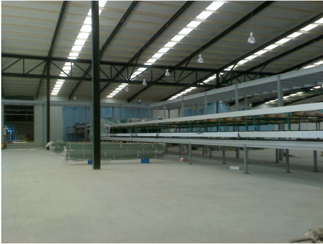
20.000 m 2 concrete based flooring 15 cm with metallic fibres Eurosteel 50/100 with Delta Joints and QUALITOP HP solution.
