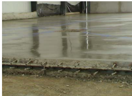
20.000 m 2 concrete based flooring 15 cm with metallic fibres Eurosteel 50/100 with Delta Joints and QUALITOP HP solution.
